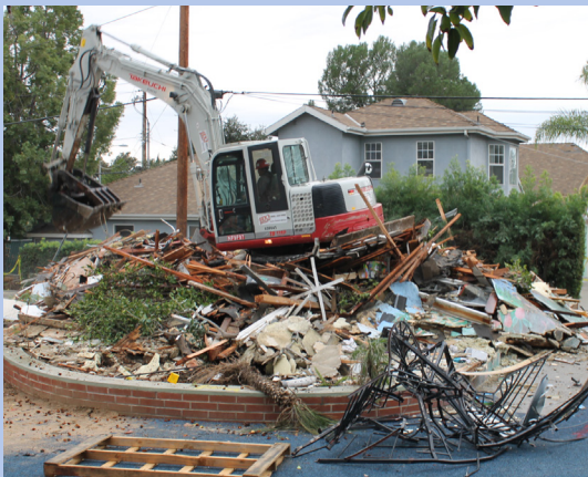
Demolition of the old buildings.
